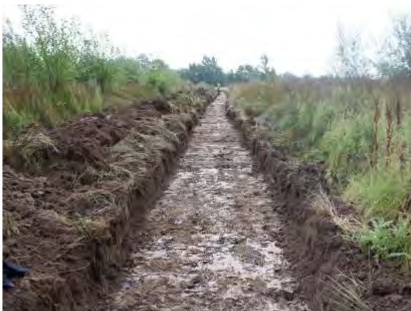
Plate 19: Trench 16, looking east
