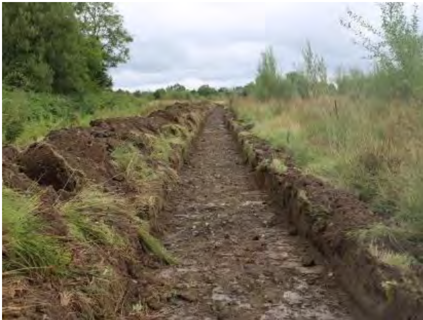
Plate 21: Trench 18 looking east
